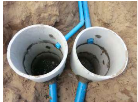
Septic Tank (Under Construction)
