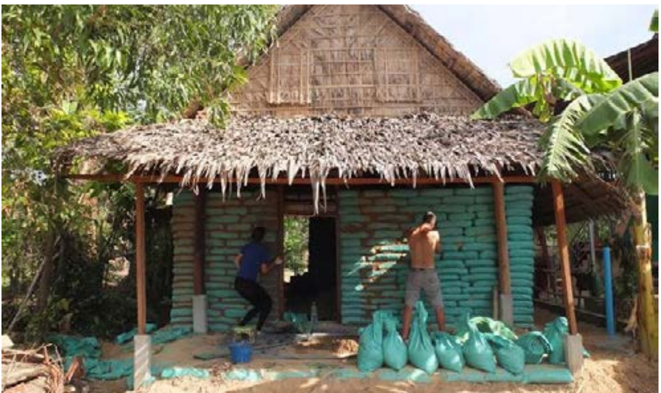
Mixing traditional Khmer features of the palm tree leaf weave roof with the earthbag technique
