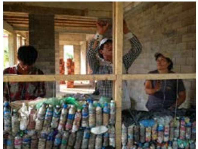
Eco-bricks constructed using plastic bottles are used to construct the walls
