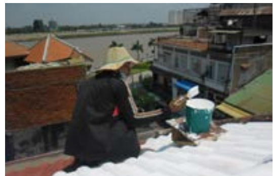
Red shingle roof in Phnom Penh is painted white
