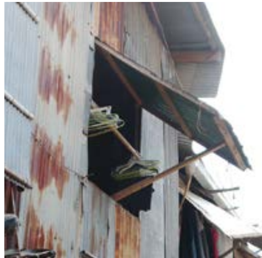
Opening with large window overhang in Sen Seak
