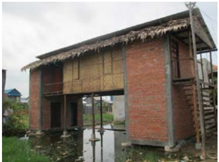
A new take on the traditional stilt house creates a shaded flexible space underneath to allow different uses during wet and dry season
