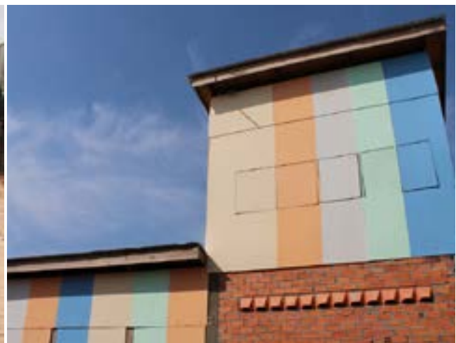
Brick walls with ventilation openings provide increased resilience.
