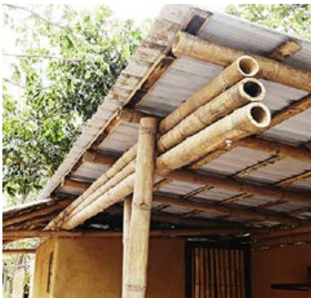
Bamboo trusses are used to form the roof structure
