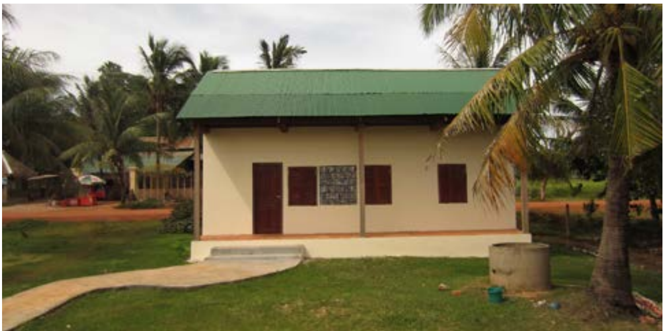
The walls of bottles are covered with plaster.
