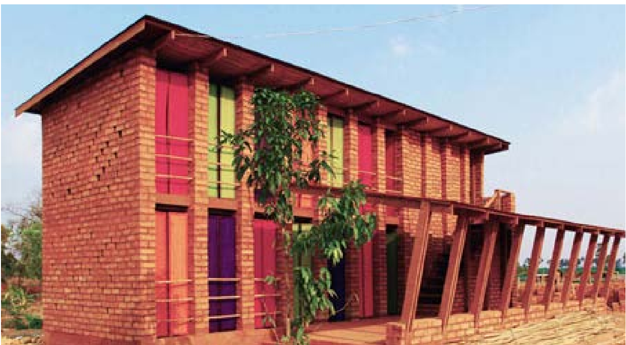
The school building is made out of local materials with local workforce. The whole community space can be opened, providing comfortable shaded outdoor space
