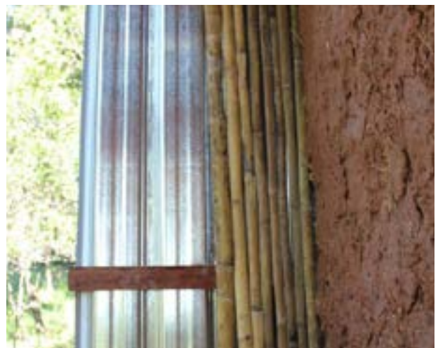
The adobe and lime plaster has a cooling effect creating a natural airflow throughout.
