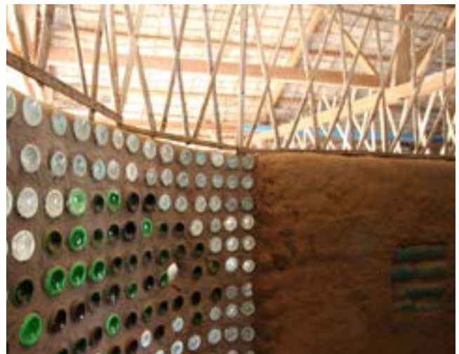
Recycled glass bottles walls can create interesting light effects in interior spaces
