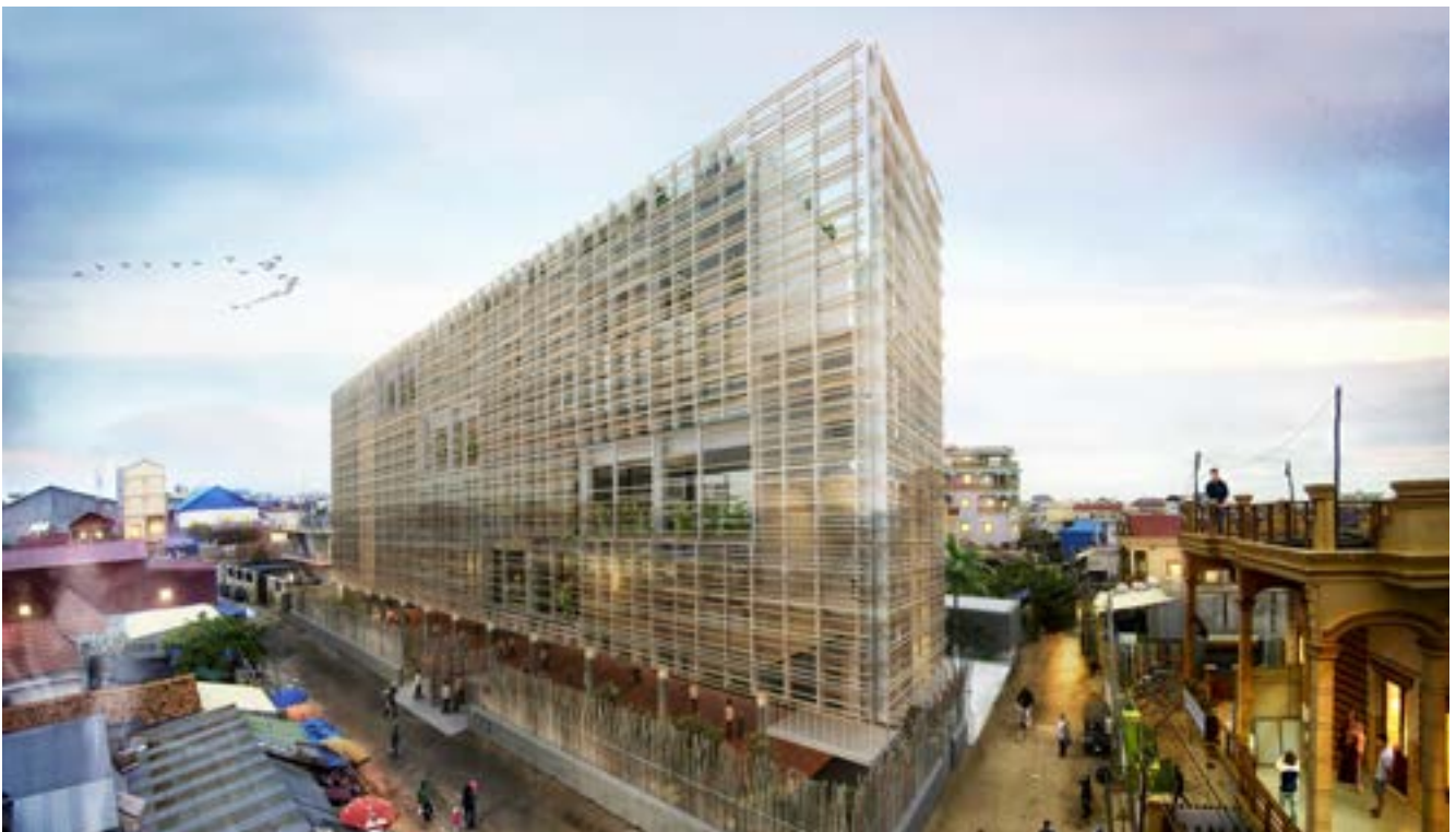
The roof top has a multi-purpose athletic court, and a teaching garden filled with local plants and vegetables, which will also help to reduce storm water runoff and minimize solar heat gain
