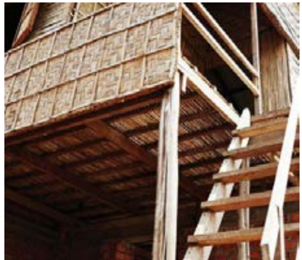
The raised structure provides shade and space for motorbikes and hammocks underneath
