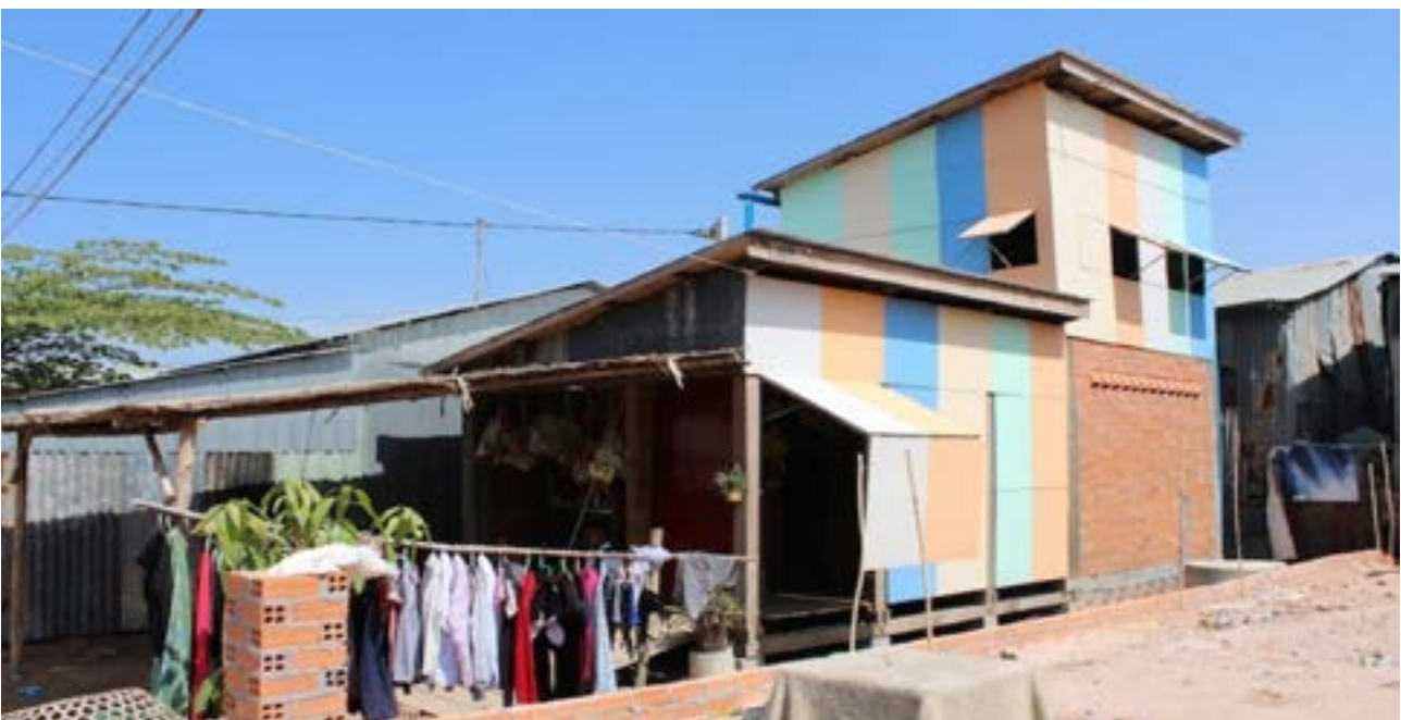
The dual-purpose porch serves as a store-front, and keeps the sense of community alive by opening the home to neighbours. Replaceable wall panels with open-able windows to allow for flexibility and privacy.
