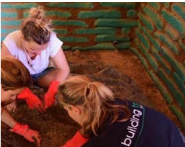
Filling the bags with earth on site
