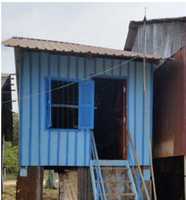
Large openings in building facade to ensure good ventilation in Roluos Cheung Aek Community
