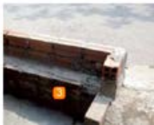
3. Shafts for flooding protection (Hesse et al., 2011)
