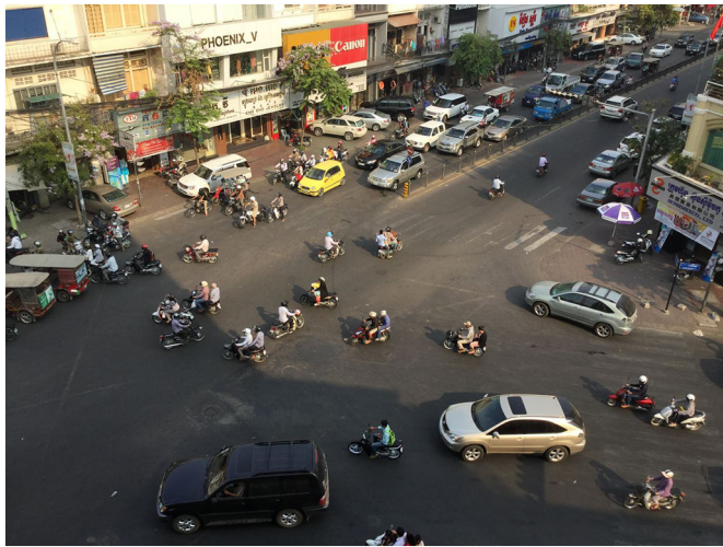
Fig. 5. Unruly status of intersection before project.
