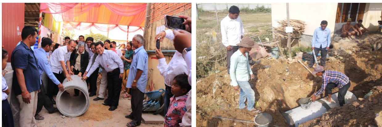
Drainage installment in low income community in the outskirts of Phnom Penh
