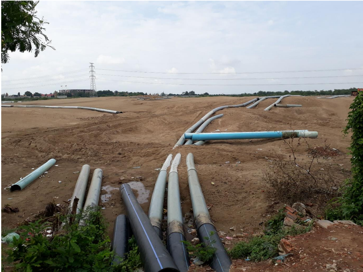
Figure 6.2 Sand Deposited through Pipes fills Boeung Tompun Wetland
