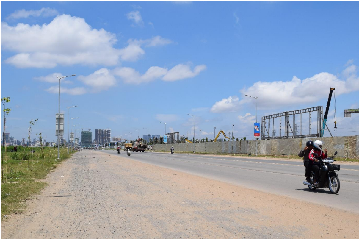
Figure 5.6 Developments going up alongside Hun Sen Boulevard
