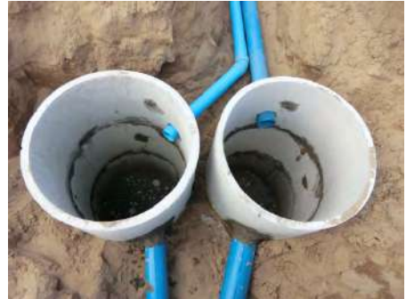
Septic Tank (Under Construction)
