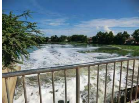
Discharged Water from Kop Srov Pumping Station
