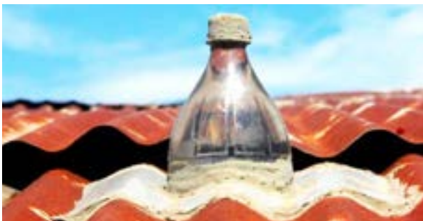
Solar bottle light in metal roof
