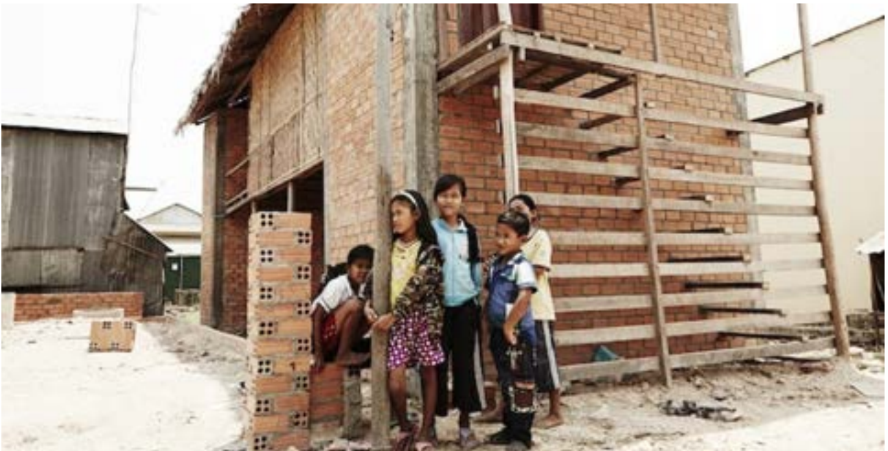
Between the columns, an enclosure is wrapped in bamboo panels, with one end opening to a raised courtyard space via swinging partitions enabling a family to extend or reduce living quarters as needed throughout the day
