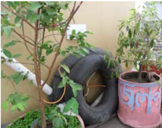
Biogas plant in Bangladesh made of Tire Tubes
