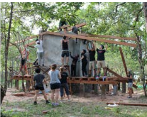
The overhanging split roof is angled to reduce solar gain on the walls.
