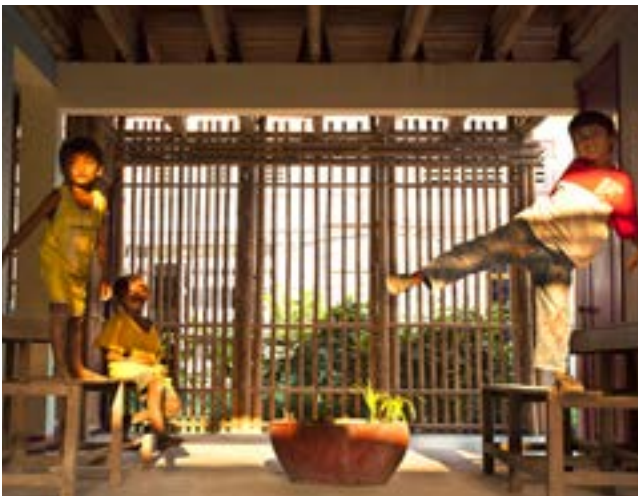
The main feature is the slatted bamboo facade, which creates a dynamic light and shadows
