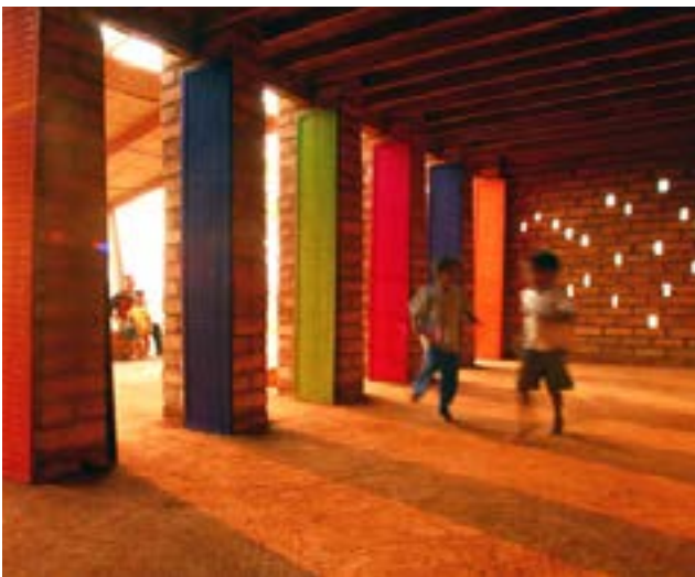
The soil block walls are laid out with small holes, for indirect sunlight and gentle wind to cool the spaces
