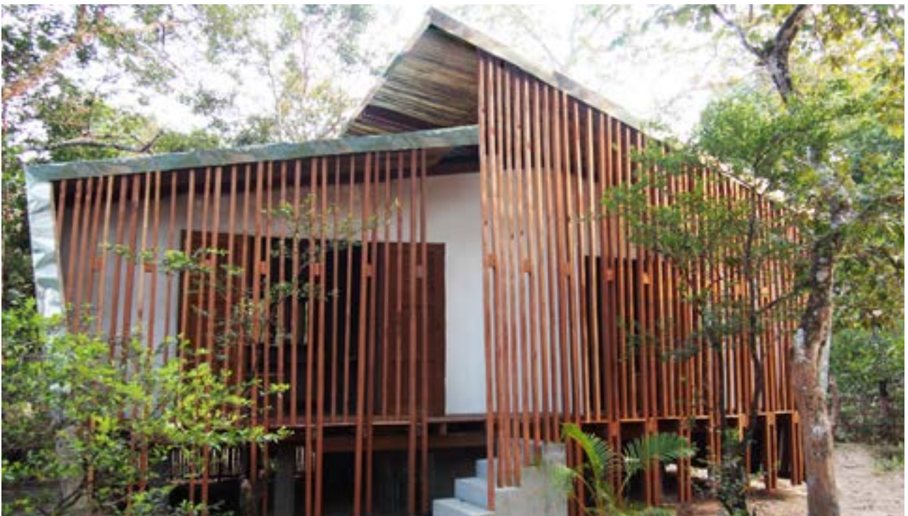
Moveable swinging windows built from locally sourced timber can be positioned to allow guests to watch wildlife
