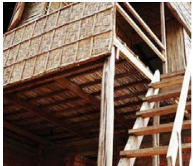
The raised structure provides shade and space for motorbikes and hammocks underneath
