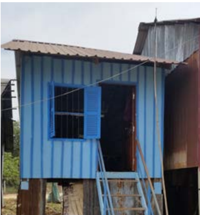
Large openings in building facade to ensure good ventilation in Roluos Cheung Aek Community
