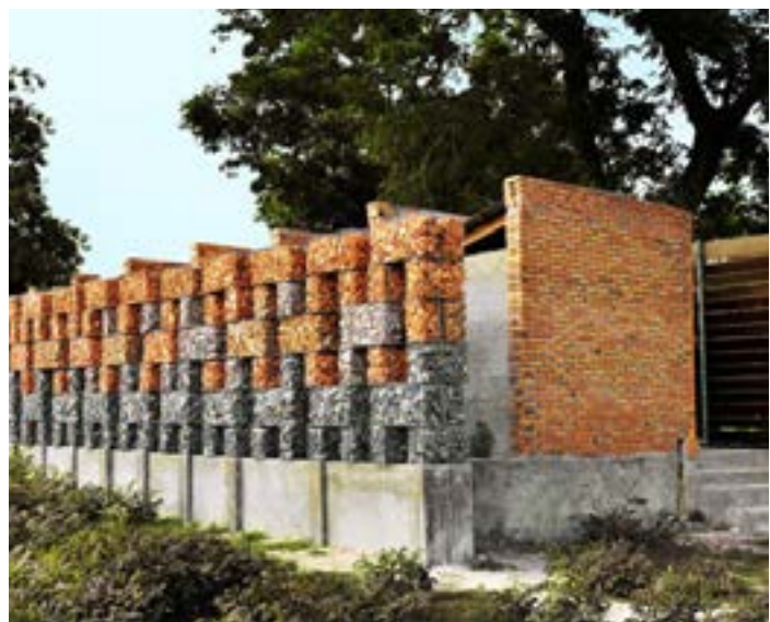
Rubble was collected from local temples that had been destroyed to create the gabion walls for the sanitary facilities.
