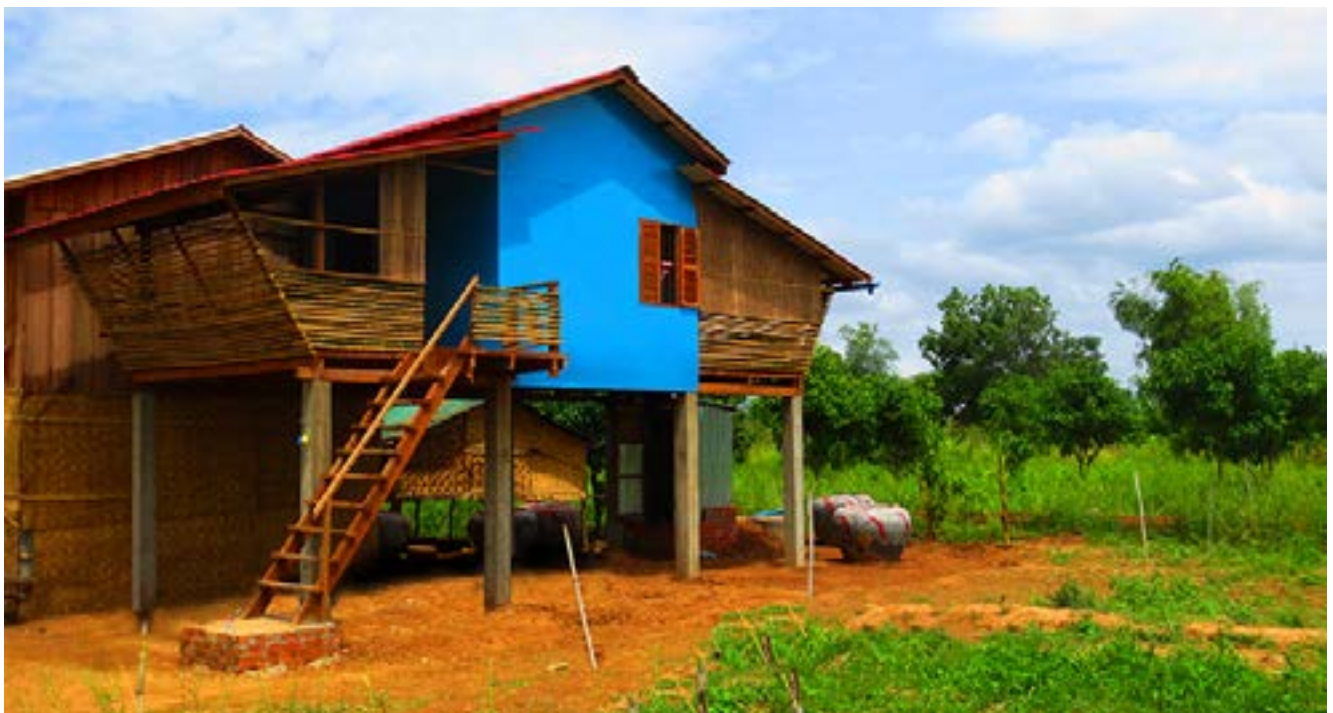
The design builds on traditional techniques and forms with a raised first floor for flood protection.
