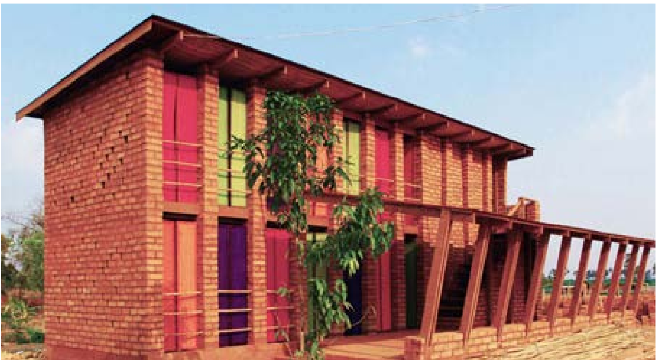
The school building is made out of local materials with local workforce. The whole community space can be opened, providing comfortable shaded outdoor space
