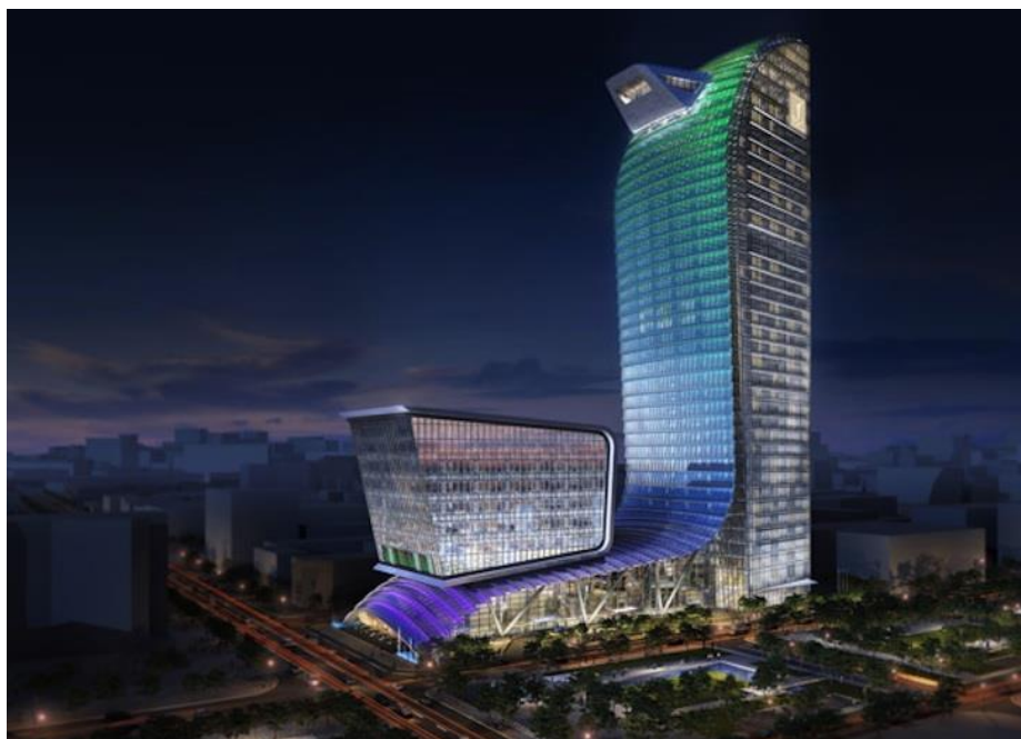
Figure 12. Energy Efficient Building in Phnom Penh
