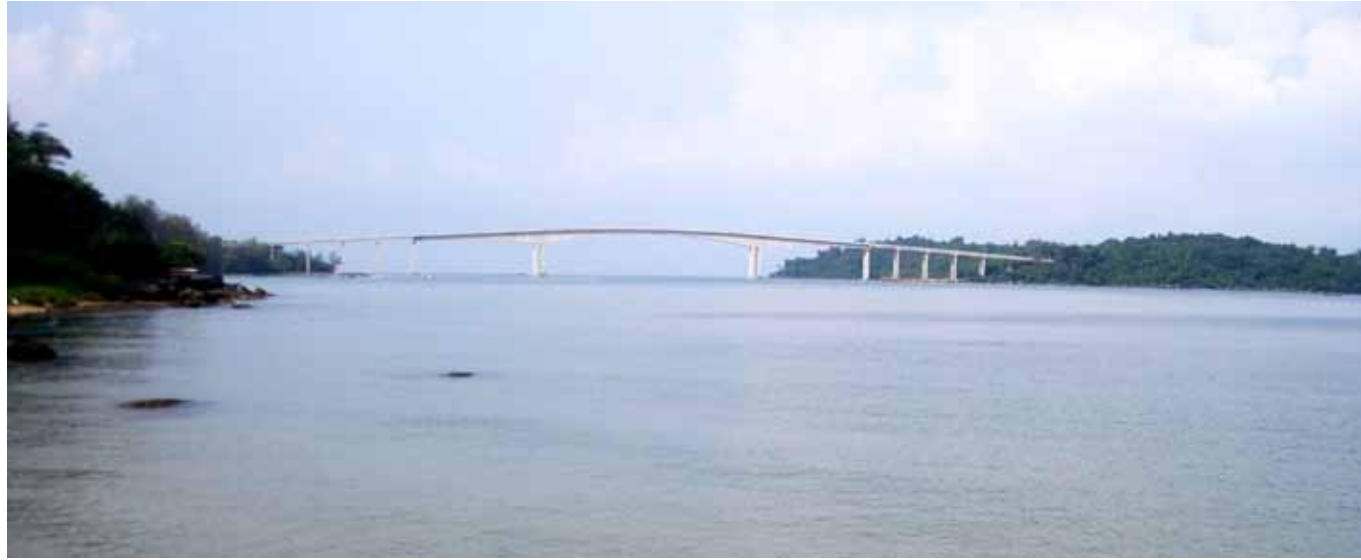
Figure 18: The impressive (and as yet unopened) Koh Puos Bridge (Above) and Thai Boong Rong's housing development (on following page) are symbols of the substantial but largely uncoordinated development in Sihanoukville
