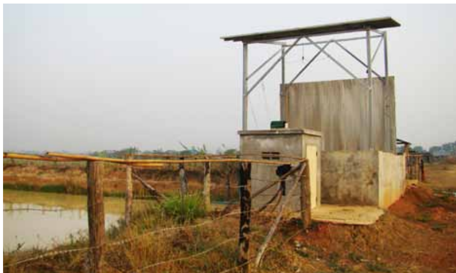
Figures 8 & 9: The relocation site (below) for families impacted by the AusAid/ADB funded railways project has been poorly managed, leaving many families struggling with inadequate and unserviced water supply (right)
