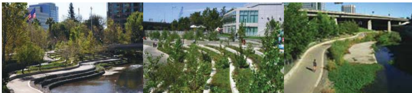
River Bank Terracing and Vegetation as Part of a Green Infrastructure Network in Guadalupe River Park in San Jose, California, United States
