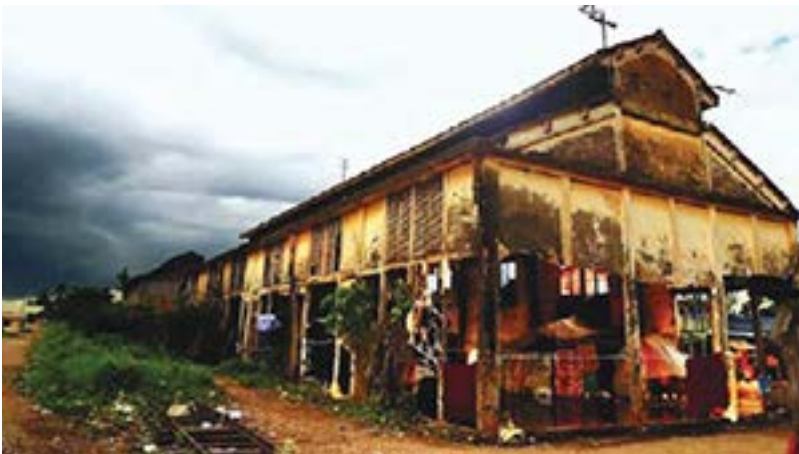
The rail yards and maintenance buildings
