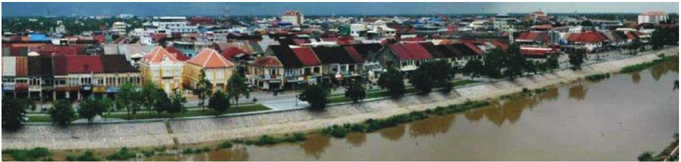
Government funded embankments on the western side of the Sangkae River
