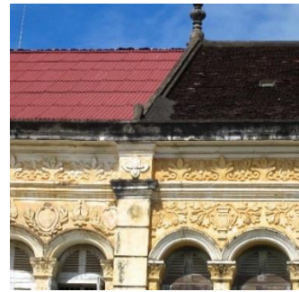
Figure B12. Contemporary (galvanised iron) and French colonial tile roofing
