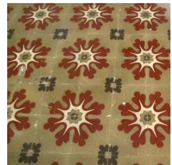
Figure B9. Floor tiles in Governor's residence
