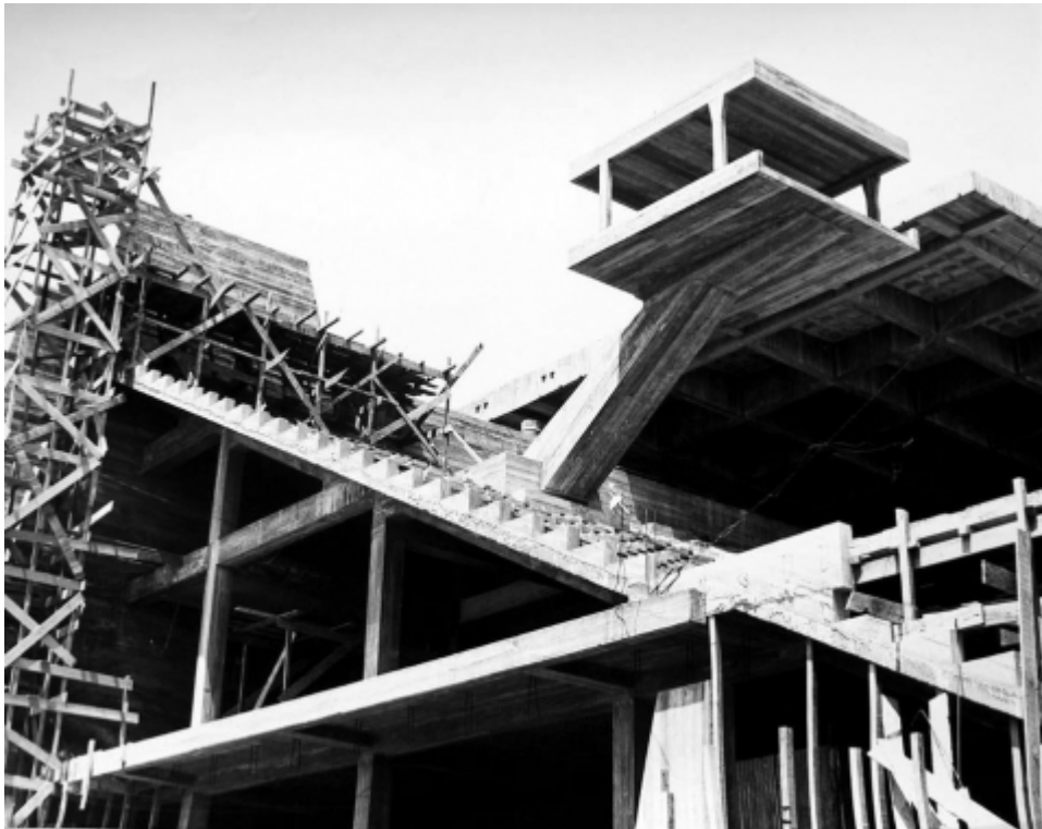
Figure 4: The National Sports Complex during construction, 1963.
