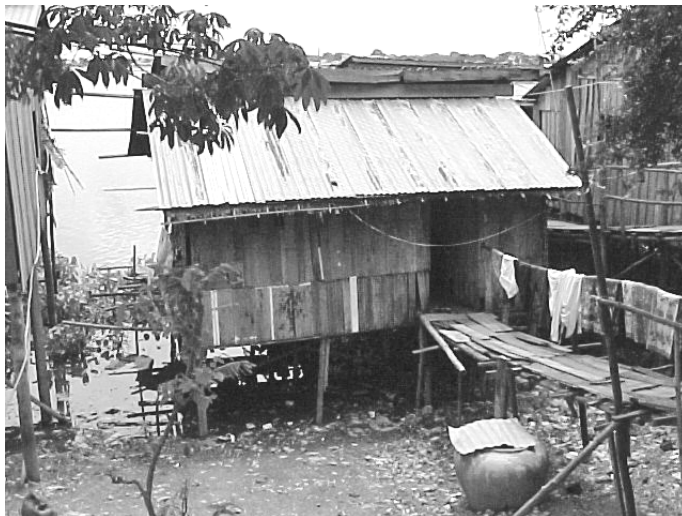
Living above a sewage pond
