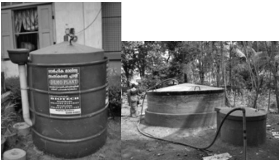
Figure 3.15 Floating drum digester tanks used in India
