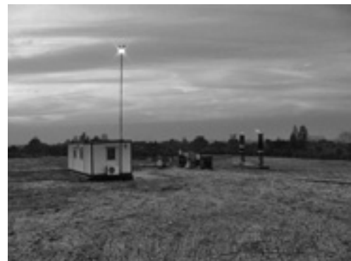
Figure 3.3 Sanitary landfill with gas recovery system in Thailand (Photo: Komsilp Wangyao)
