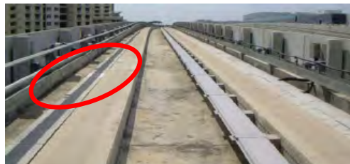
Figure 3.5-6 Image of Contact Line of AGT
