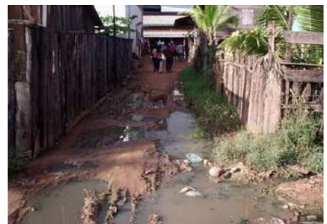
BEFORE : (above) This is one of the roads in the Samrong Thmey community, before upgrading.
