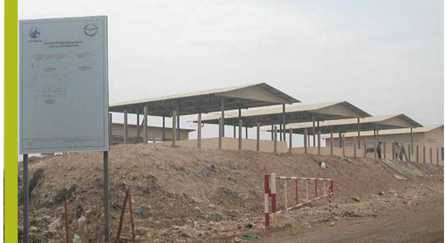
The waste pickers' multipurpose center, built by the project, at the municipal dumpsite.
