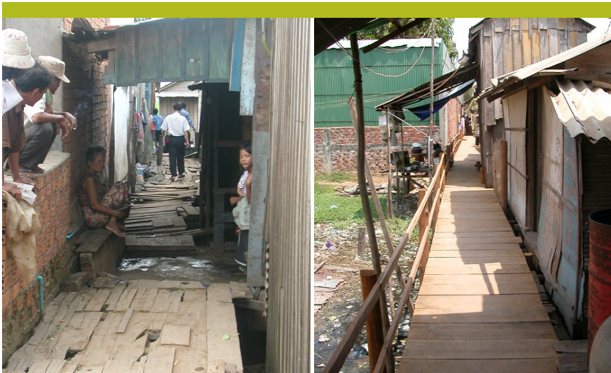
Footbridge construction. Before (left): Unsanitary conditions underneath the wooden houses and inaccessible walkways pose health risks and hazards. After (right): A wooden footbridge was built, greatly improving living conditions. Location: Psar Daeum Thkhov.
