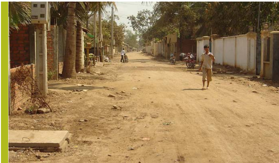
Poor roads are difficult to access during the rainy season and dusty during the dry season.
