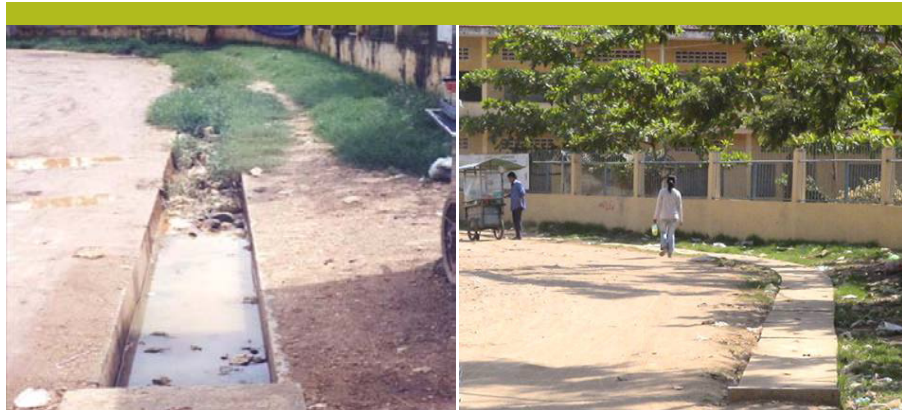
Drainage rehabilitation. Before (left): The open unmaintained drain was a huge eyesore. After (right): The drain was cleaned, repaired, and concrete covers were put in place. The drain is functional, and the school (right) planted grass to beautify the surroundings.
