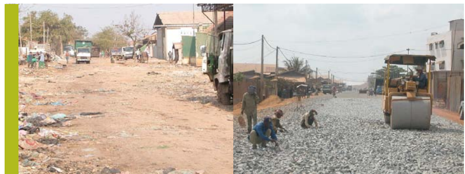
Access road to the municipal dumpsite, before and during construction.
