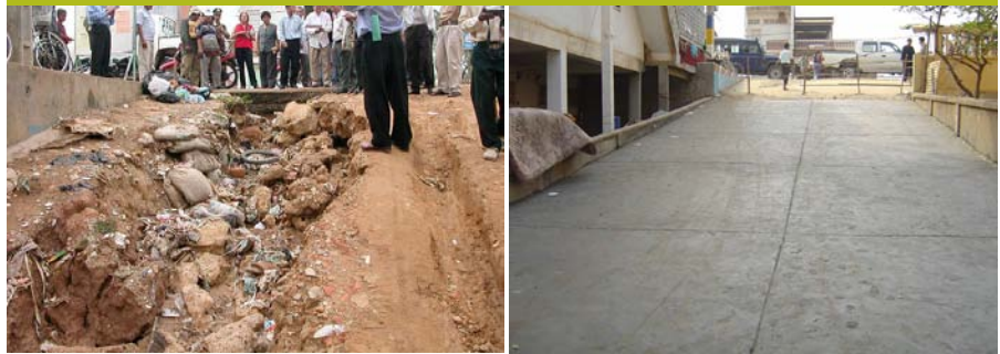
Concrete road pavement. Before (left): Huge gaps and erosion were dangerous for pedestrians and vehicles. This road was impassable during the rainy season. After (right): Bamboo-reinforced road surface pavement improved the roadway's function and appearance. Location: Boeung Tumpon.
