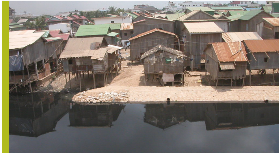
Poor drainage is not only detrimental to the city's visual environment but to public health as well.
