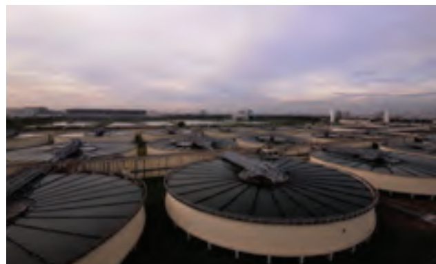
A water treatment plant
