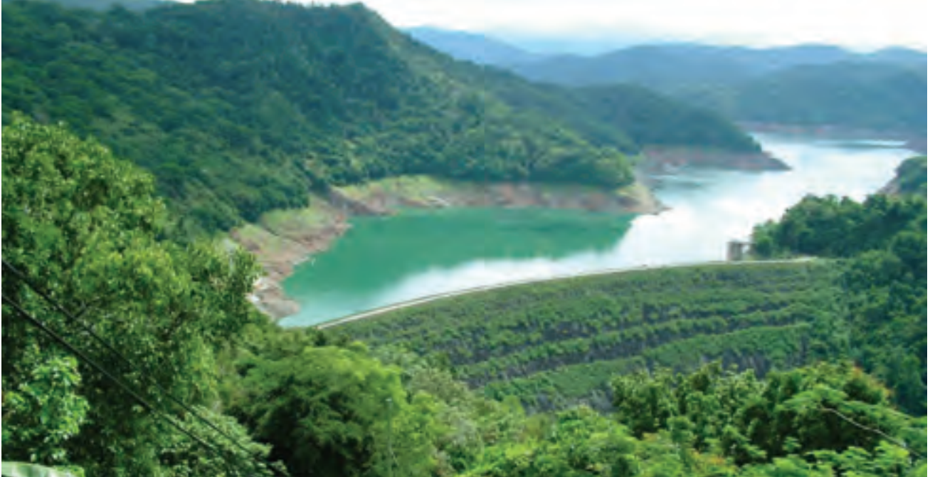
Water source at Angat Dam, Bulacan, Philippines
