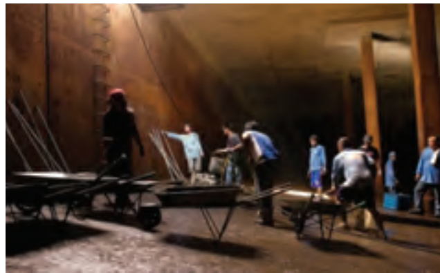
Cleaning and disinfecting the reservoir
