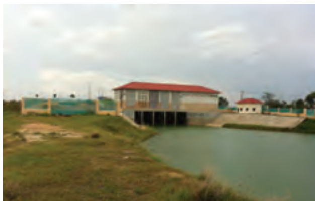
Open-canal source of water
