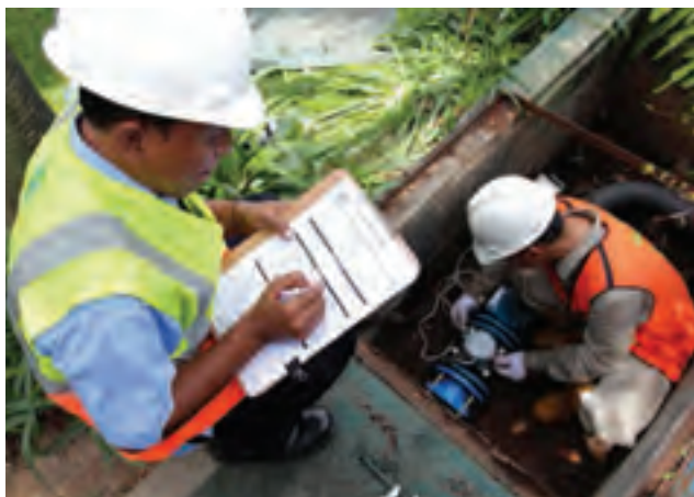
Reading a water meter to control nonrevenue water
