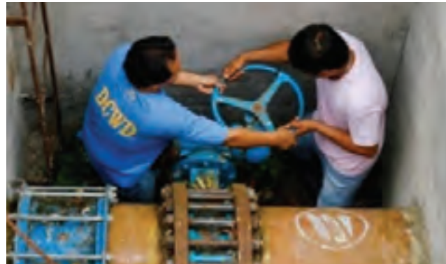
Valve turning for distribution
