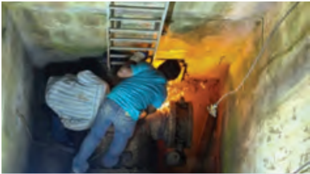
Installing a 600 mm butterfly valve
