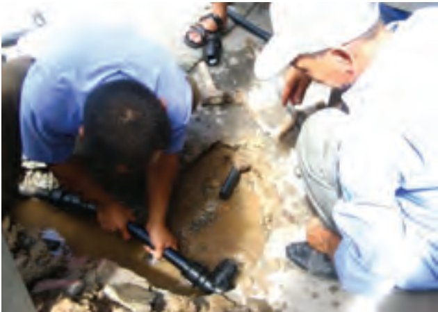
Repairing a leak
