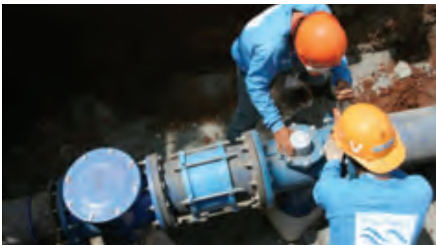
Repairing a distribution leak (a)
