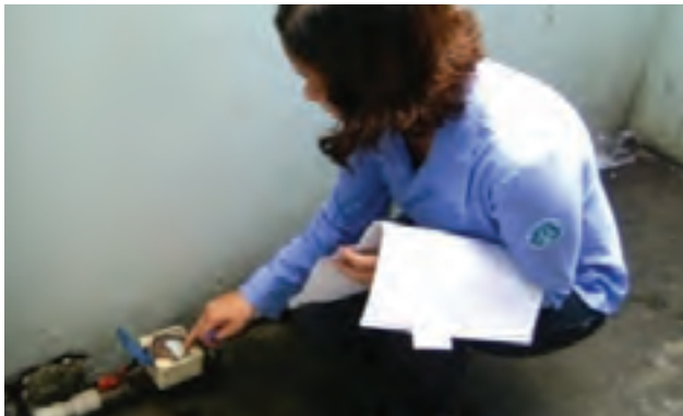
Reading the water meter
