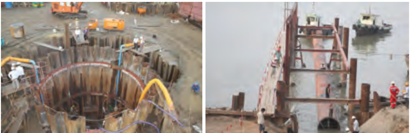
Constructing a water intake
