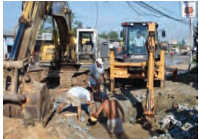
Repairing a broken water distribution pipe
