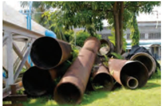
Old corroded pipes
