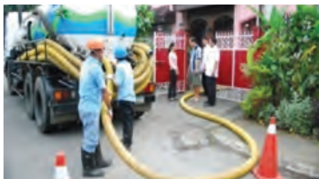
Septic tank desludging
