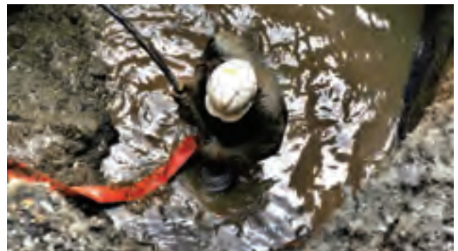
Repairing a distribution leak (b)
