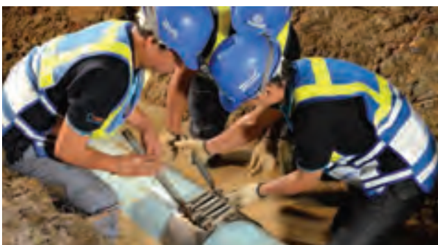
Repairing a distribution leak (e)
