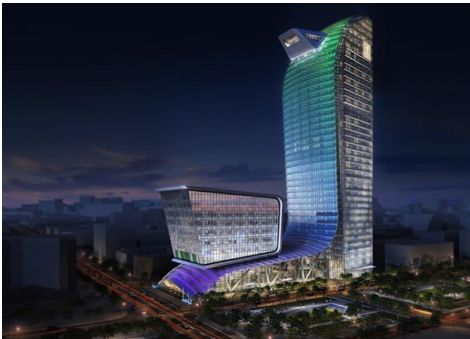
Figure 12. Energy Efficient Building in Phnom Penh
