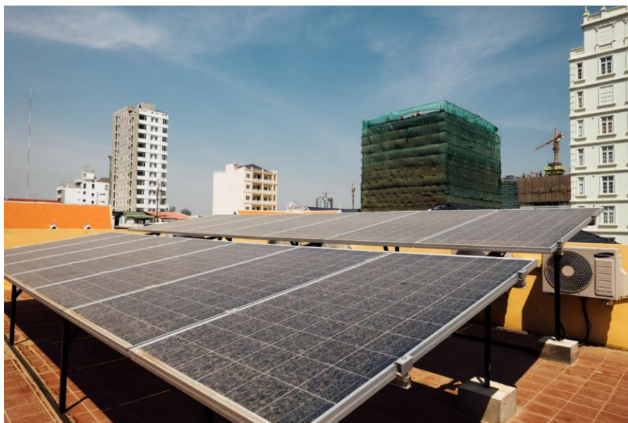
Figure 10. There is substantial potential for roof-top solar PV in Phnom Penh to service households, businesses and manufacturing (photograph by Bernardo Salce).
