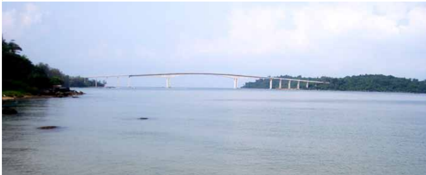
Figure 18: The impressive (and as yet unopened) Koh Puos Bridge (Above) and Thai Boong Rong's housing development (on following page) are symbols of the substantial but largely uncoordinated development in Sihanoukville
