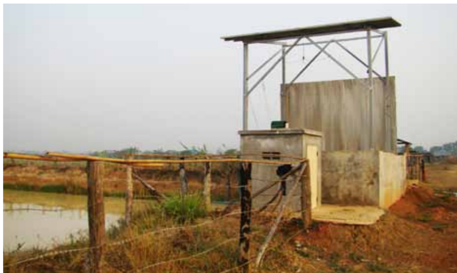
Figures 8 & 9: The relocation site (below) for families impacted by the AusAid/ADB funded railways project has been poorly managed, leaving many families struggling with inadequate and unserviced water supply (right)
