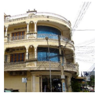
Figure B11. French colonial architecture and intrusive power lines
