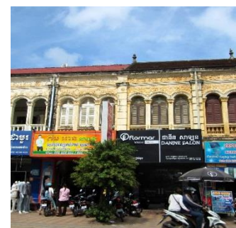
Figure B10. French Colonial architecture masked by contemporary signage
