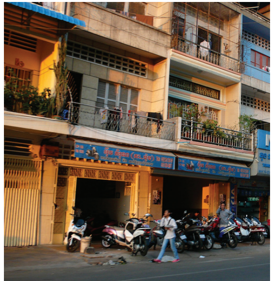
Figure 13: Typical shop houses with ground floor parking and shops and housing above. Interior living and sleeping quarters have no access to direct daylight and fresh air. Photo by author.
